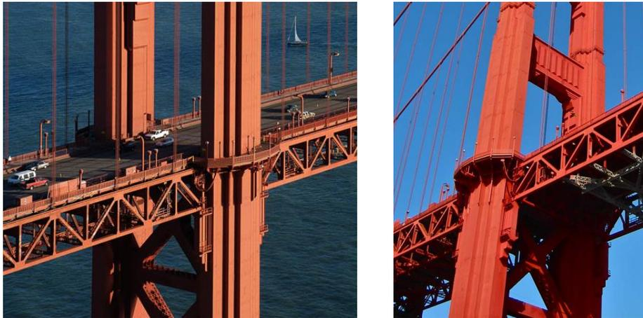
**Figure 3:** Connection of deck and truss system to pylon
